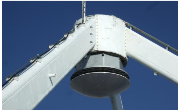
M2 installed on the tetrapod head
